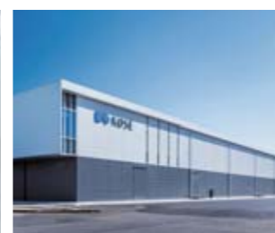
New manufacturing facility at the Gunma Factory
